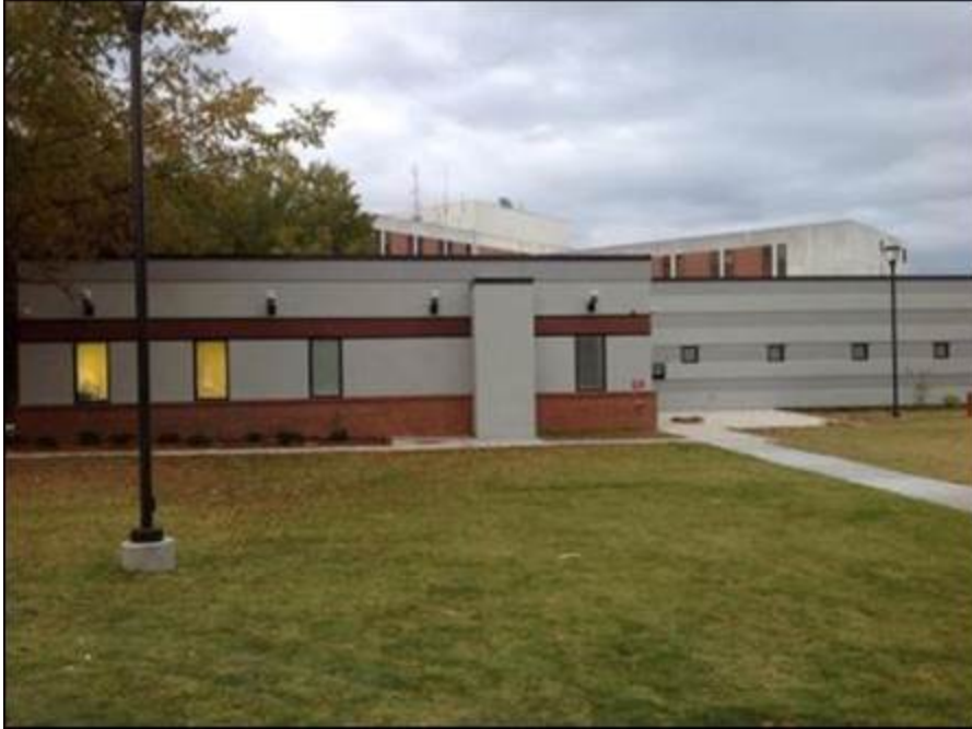
New Freedom Health Center well underway toward completion. This will be a major boon in caring for returning service members. VA Photo/Kevin Lee McIver
